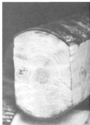
PLATE 63 The two sides hewed, the log is now ready for notching. The remainder of the sides will be hewed after the logs are all in place in the cabin.
