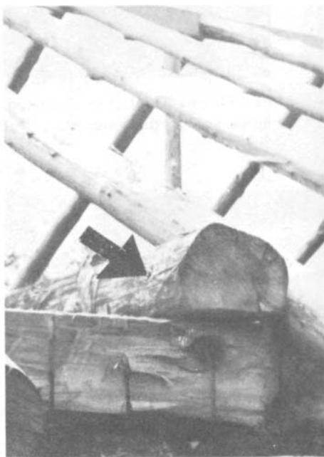
PLATE 98 Note how the joist (arrow) is left round except for the lap joint cut to fit the plate.
