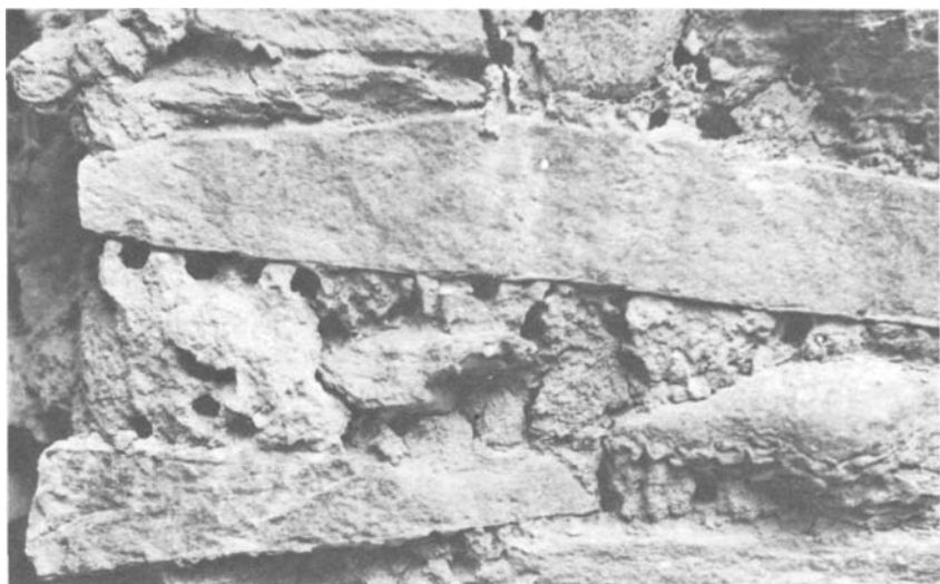
PLATE 144 A common problem with all-mud chinking was that it soon became the home for bees as the holes in this chinking show.
