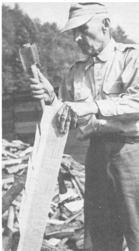
PLATE 32 Bill prefers removing the sap from the finished shingle since the sap is softer and rots quickly when exposed to the weather. Some place the sap edges together on the roof and cover them with a third shingle for protection.
