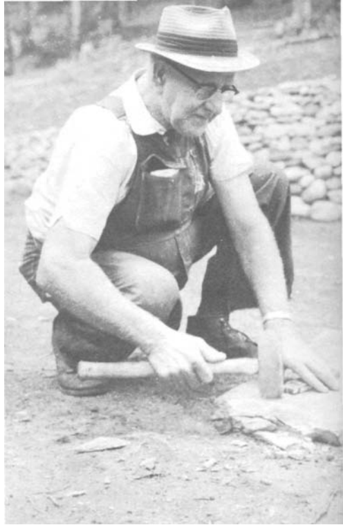
PLATE 149 Often the flagstones must be reshaped to fit. Claude measures the hole to be filled and then breaks the excess away with a hammer.
