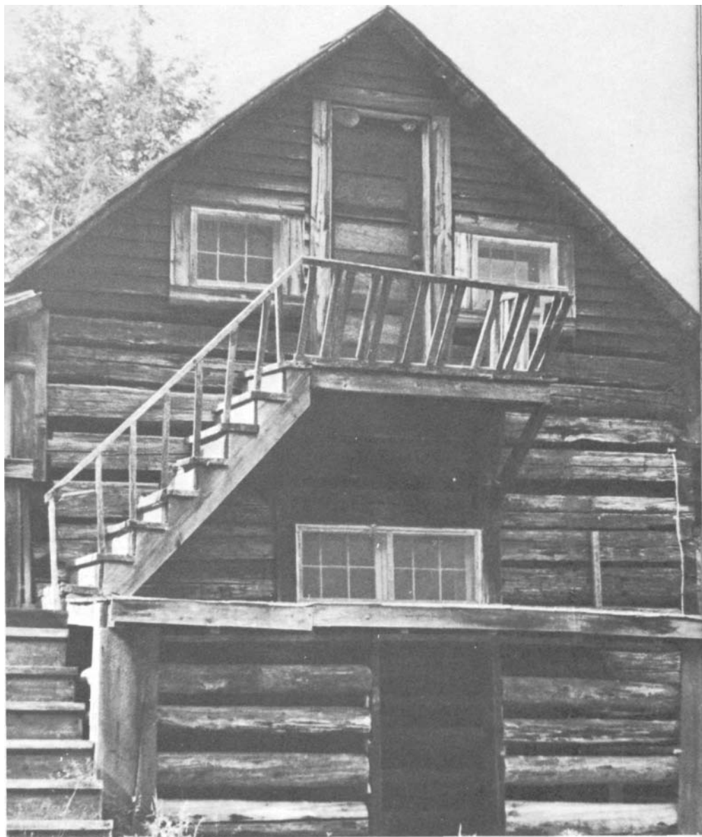
PLATE 123 The gable can be designed to hold a door and windows, as seen on this cabin at the Jay Hambidge Art Foundation in Rabun County.
