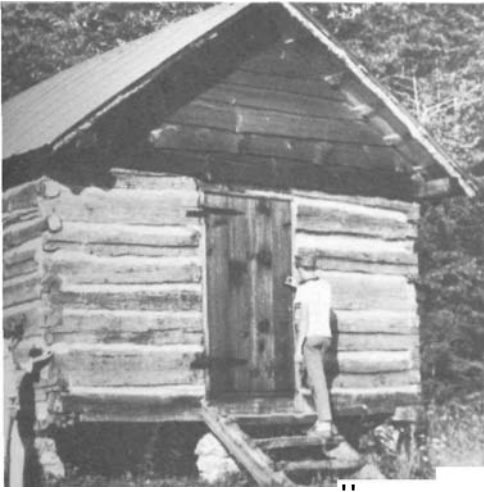
PLATE 120 Richard Page and Robbie Letson examining a windowless house with a board gable. Arrow points to joist.
