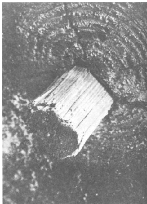
PLATE 134 A locust peg over two hundred years old in the hole it was cut to fit.
