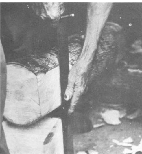
PLATE 68 Now, placing the ruler as shown, draw a vertical line on the top log which intersects with the sloping line.
