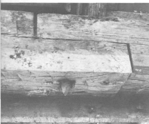
PLATE 92 Two logs were hewed and lap-jointed together to make this plate. A wooden peg through the joint ensures that they will not slide apart.
