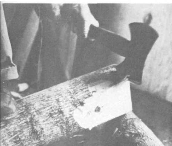
PLATE 64 Slope the top surface at a 30-45° angle
