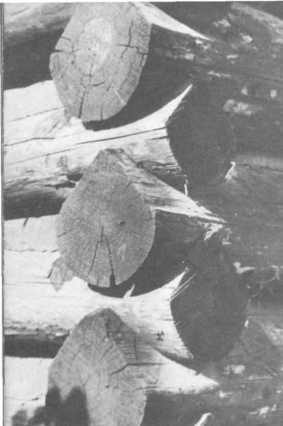
PLATE 83 Here's how the corner should look if you followed Hillard Green's method . . .
