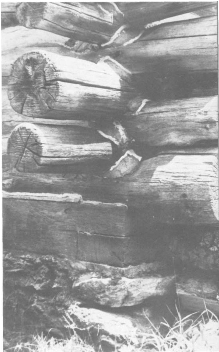
PLATE 60 The lap joint of this end log (arrows) fits snugly over the sill.
