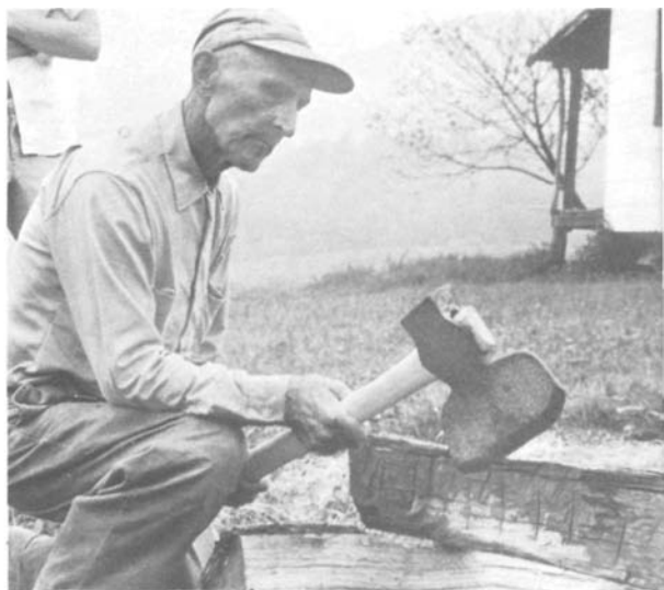
PLATE 15 Bill Lamb shows how to use a broadaxe. The vertical marks on the log were left by the scoring process.
