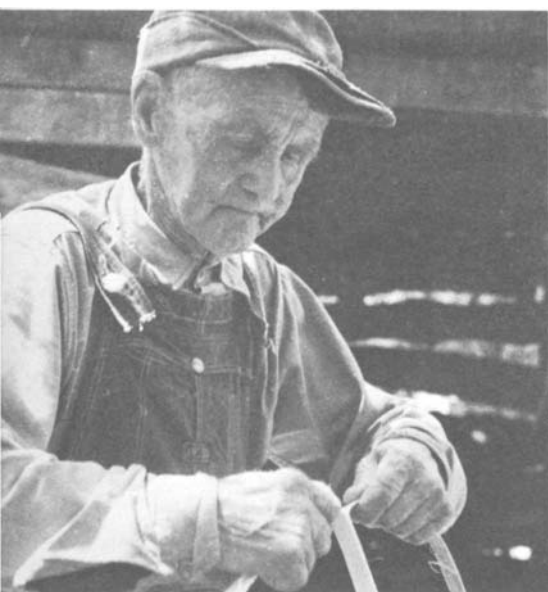
PLATE 156 Continue in this same fashion with each succeeding slice until the splits are the desired thickness.
