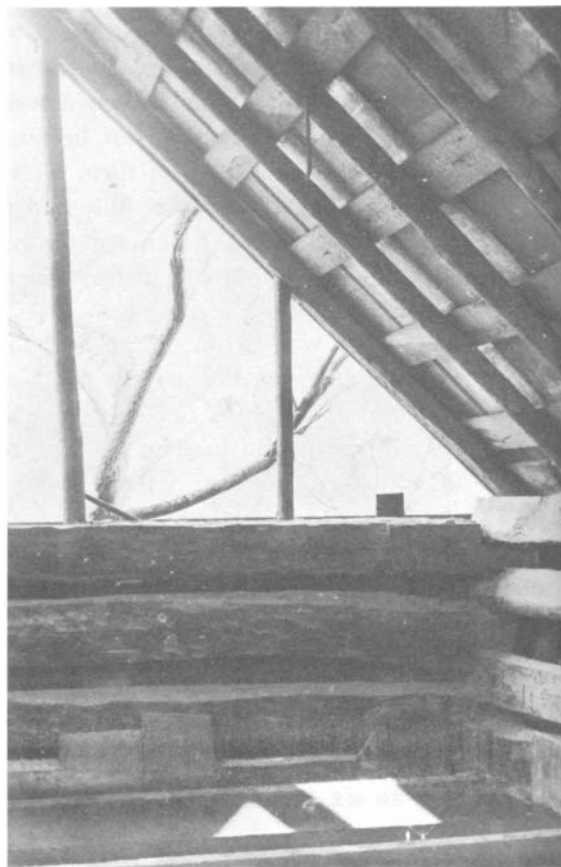
PLATE 106 The ends of these rafters are sloped and set directly on the last wall log. Note also the lathing for the roof.
