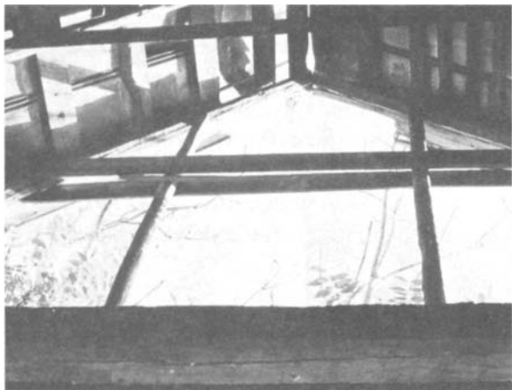
PLATE 118 Poles can be used as the gable's vertical supports.
