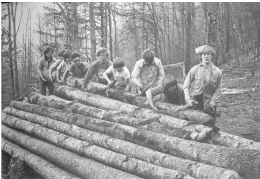
PLATE 360 When Wig was building his log cabin, we all went out and helped cut and drag the poplar logs up to the foundation. We made a real party out of an otherwise tough job.
