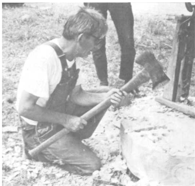
PLATE 140 Working only on those four buckets that cut across the grain, Sam roughs out the buckets with an axe and . . .
