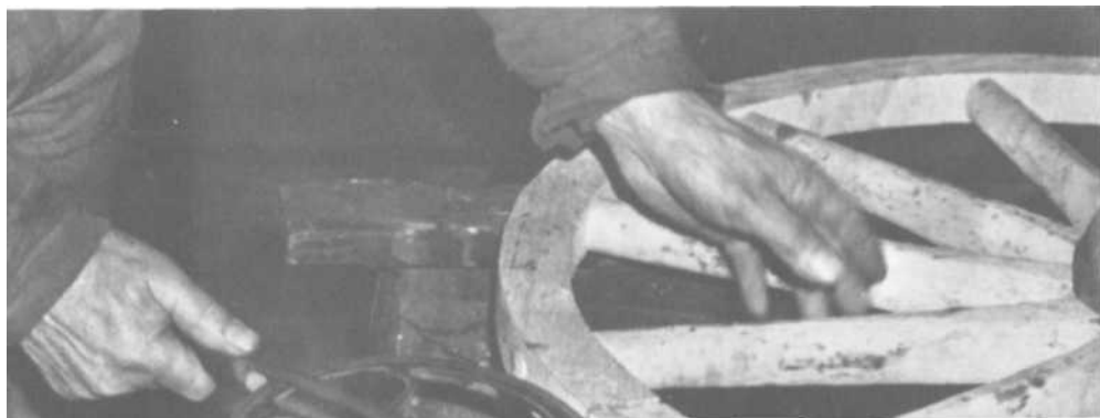
PLATES 105-106 With a traveler, John checks the circumference of both the wheel and the metal "tire" to make sure the fit is good. The tire should be about a half-inch smaller in inside circumference than the outside circumference of the wheel itself. This insures a tight fit.
