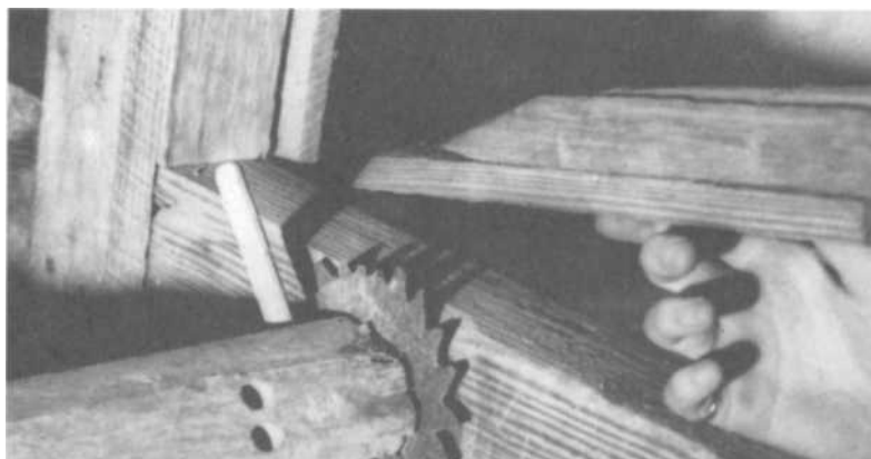
PLATE 284 Cog end in place. See also Plate 289 .
