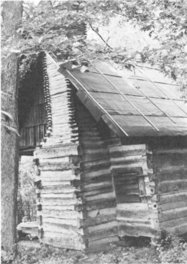
PLATE 372 A beautiful stick-and-mud chimney on a cabin near Brasstown, North Carolina. Note also the gable of hand-split shingles and the wooden shutter with wooden hinges covering the window. Such shutters were used in place of glass, which was not available at the time.
