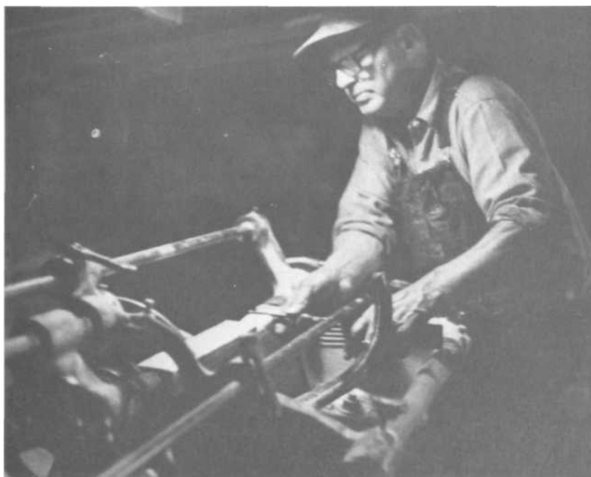
PLATE 84 The spokes were turned on a pattern lathe. Years ago, they would have been carved out with a drawing knife.
