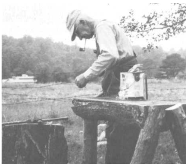
PLATES 320-322 Mr. Dickerson notches the ends of the three legs to fit the battling bench, and then nails them into place. The bench has three legs so that it will set steady, even on rough ground.
