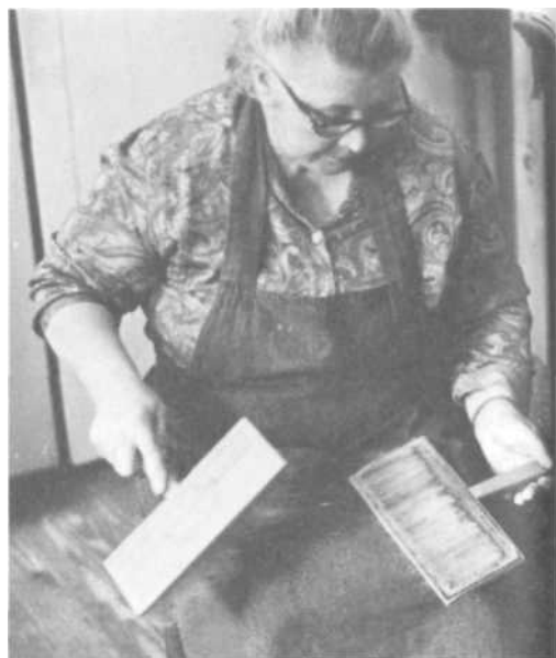
PLATES 205-207 In making rolls for spinning, Margaret uses a set of fine-toothed "roll cards." She takes one bat, pulls it apart, distributes it over the top card (Plate 205) as before, and combs the wool several times (Plates 206—207) as before (motions A and C).
