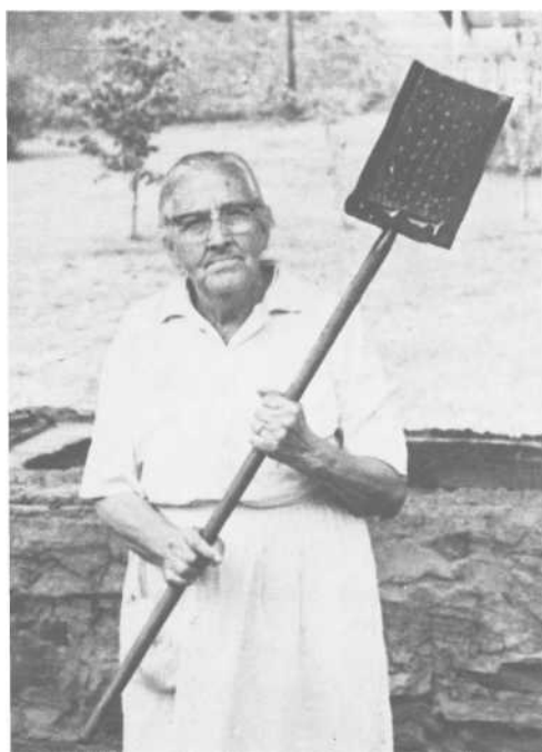
PLATE 427 Mrs. Brooks holds the skimmer. Note the holes in its bottom—juice runs through them but foam doesn't.
