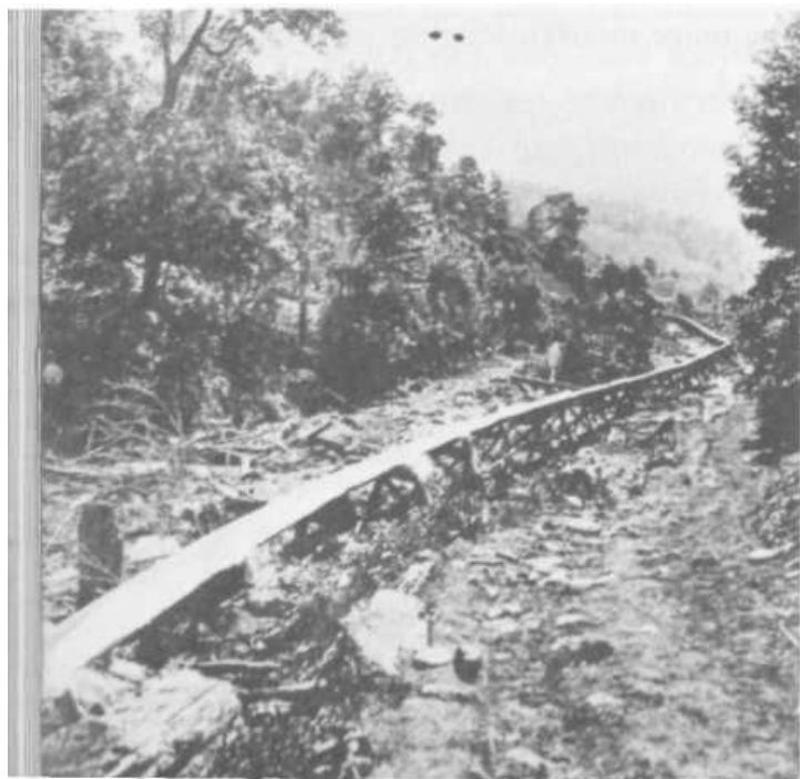
PLATE 271 Acid wood (chestnut) was essential for the production of paper. Companies like Champion International would build miles of flumes up into the mountains in order to get this acid wood out. A flume would begin high in a watershed nearly at the head of the creek. A splash dam at the head of the flume would hold water to be turned into the flume. The chestnut would be cut into five-foot lengths and split up and stacked beside the flume at intervals along its length during dry weather. Then, in wet weather when the stream was running full, water would be turned into the flume at the splash dam and the split wood would be loaded into it and carried to its end. The flume pictured here was on Big East Fork. (Photo courtesy of Champion Paper, a division of Champion International Corp., furnished by C. W. Hardin.)
