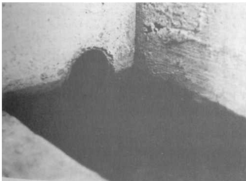
PLATE 338 Point E, view of pipe that carries water from the water inlet areas to the trough in the springhouse.
