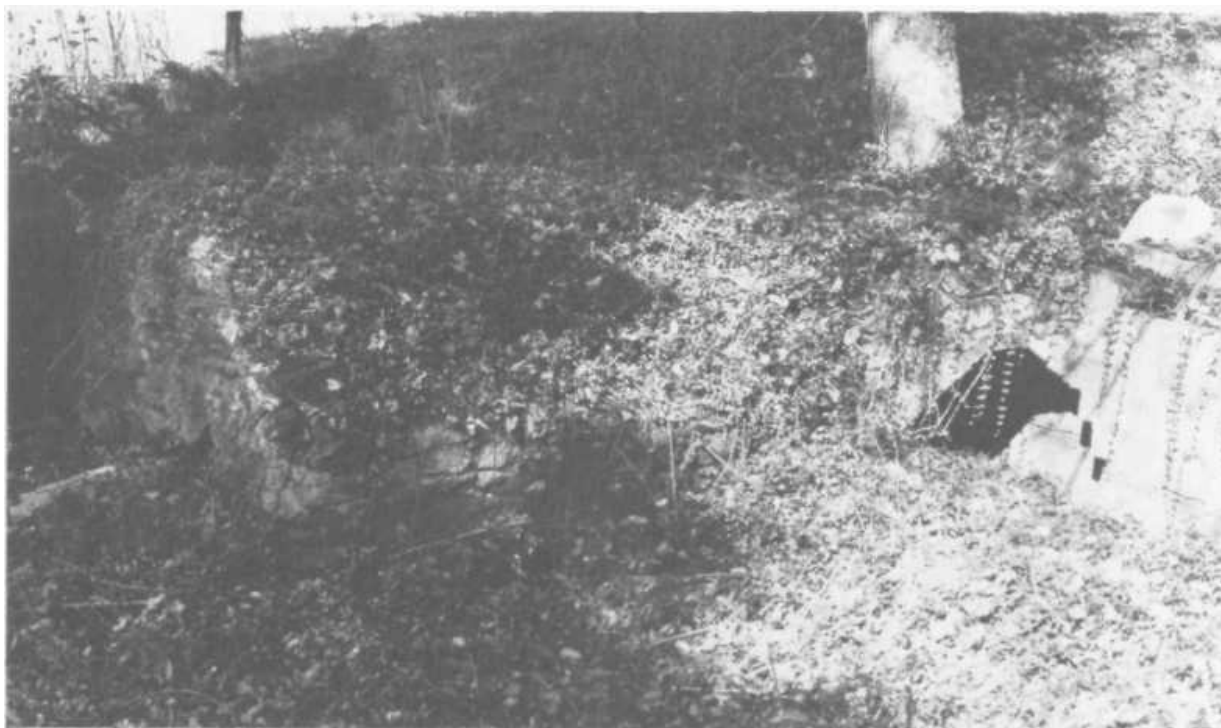
PLATE 324 Point F, overall view of the springhouse.
