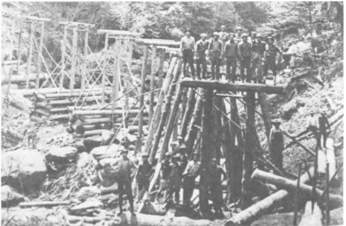
PLATE 274 Narrow-gauge railroads were also used for hauling large logs, surh as balsam, to the mill. Often trestles were required, and a man like Rube Mull and his crew would be railed in to build them. This trestle probably went up into Little East Fork, an area that is now the Pisgah National Forest. (Photo courtesy of Champion Paper.)
