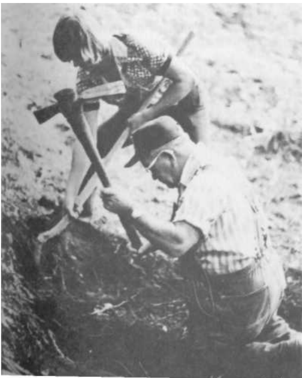
PLATE 426 The first step is to choose a suitable hillside hidden in the woods. Buck always sets his stills into a bank so that he can stand on the ground behind the still and get to it without using a ladder. The site selected, he and Joey Fountain, one of the Foxfire students, dug out the hole for the furnace.
