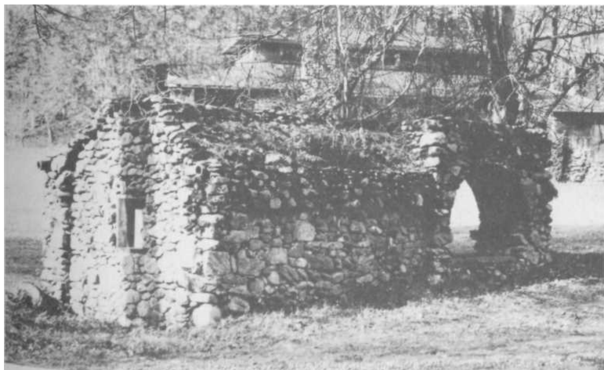
PLATE 334 Point A, view of Hambidge springhouse.
