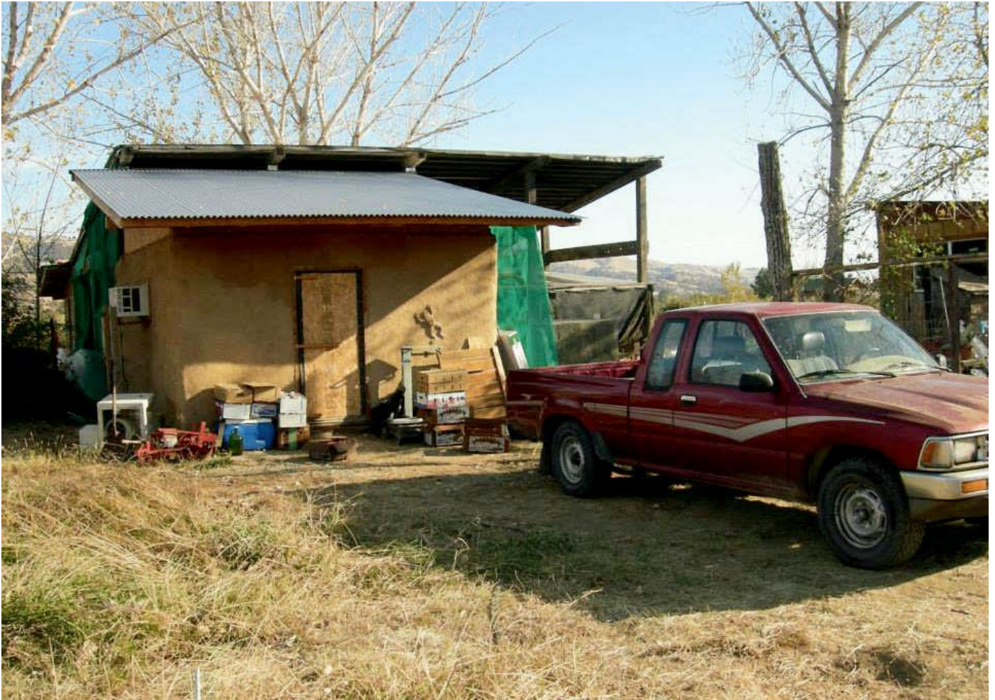
ABOVE: Annie's straw-bale cooler for produce storage
