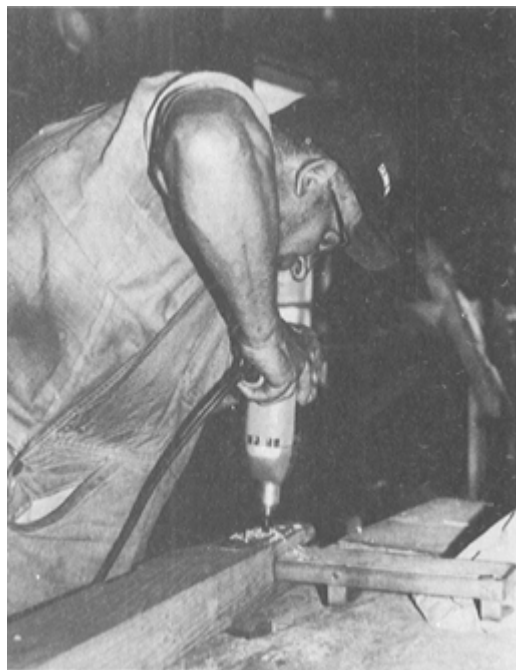
PLATE 314 ... drills a hole through each for a locking bolt, and bolts each into place.
