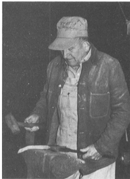
PLATE 220 Now that the hubs are banded so they cannot split, Jud finishes hollowing them out with a rounding chisel he made for this purpose.
