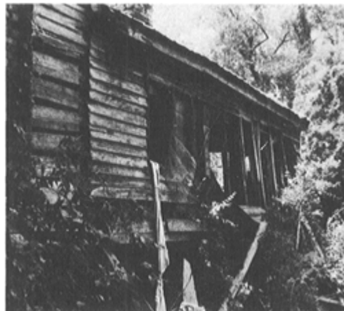
PLATE 397 The siding for the F-H addition, or the kitchen wing, was removed first.
