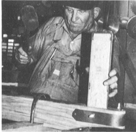
PLATE 326 Again, U bolts are used to tie the bolster, hounds, and axle together.
