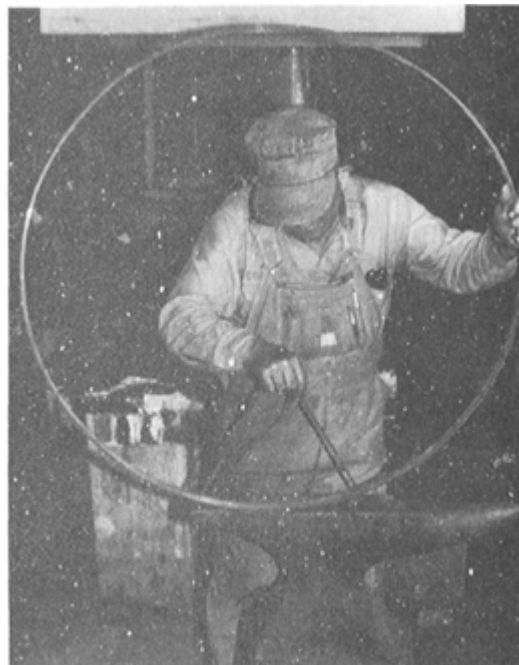
PLATE 257 Then he took a pair of dividers, the legs of which were braced by a horizontal bar to keep the legs from opening or closing during the operation. Since he wanted to shrink the circumference of the tire by three eighths of an inch, he placed one leg of the
