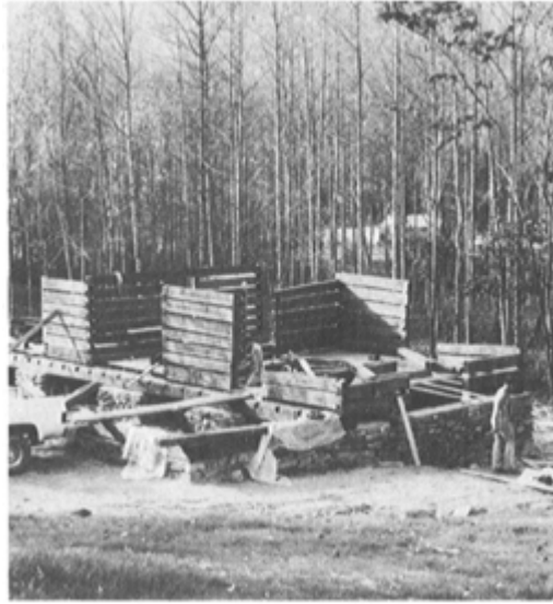
PLATE 413 The sill log diagrammed in Plate 436 is visible in this photo, set into place against the sill log for the two-story section. As the wall logs were set back into place on their new foundation, there was ample opportunity to plumb the walls again and straighten any portions that had sagged with age.
