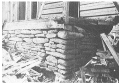
PLATE 395 Beneath the long walls of the additions and the original house were solid foundations of flat rocks mortared by red clay. The foundation work beneath the entire building was one of its most striking features, most log houses being built simply on rock pillars. All the foundation rocks were loaded onto trucks and taken to the reconstruction site.
