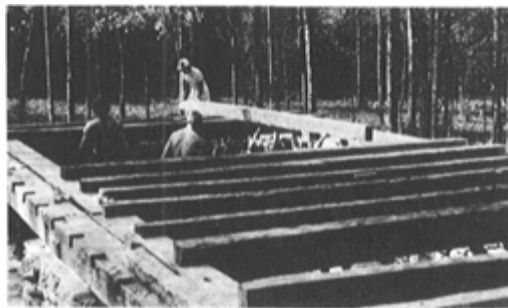
PLATE 408 Students from a Foxfire class helped former students Clay Smith and Darryl Garland set the foundation logs (sills) and floor joists for the two-story section into place first.
