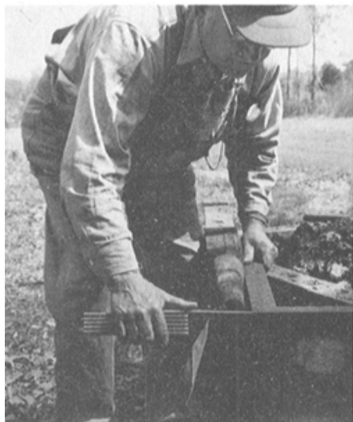
PLATE 270 Next he measured and sawed out the new axles from seasoned oak timber.
