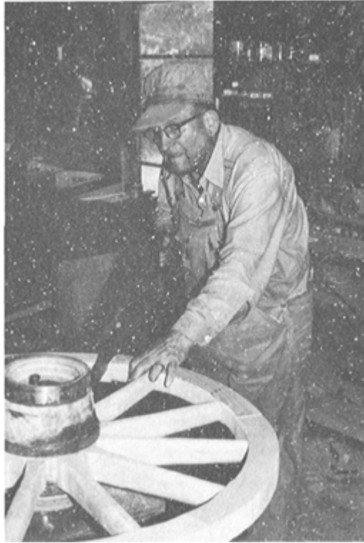
PLATE 242 As all old wagon makers did, Jud “saws the joints” between the felloes to make the faces meet properly and to create a bit of slack space for the metal tire to pull together as it shrinks around the wheel and creates dish. According to Jud, it is also acceptable to saw out a three-eighths-inch space between two felloes and leave the other joints untouched.
