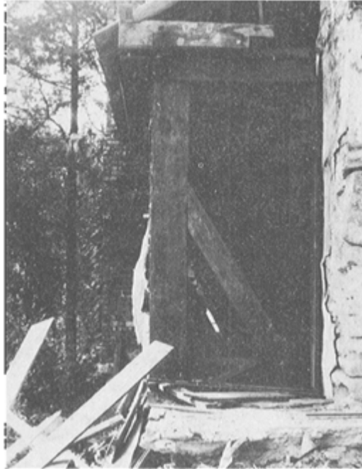
PLATE 401 The corner post beneath this point was supported by a diagonal brace ...
