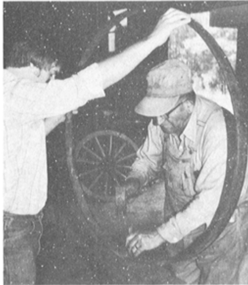
PLATE 256 Using a trick he learned from an old man he once worked with, Jud made a mark on the inside of the tire with a center punch.
