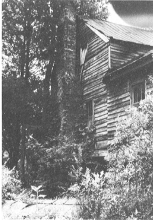
PLATE 392 The Rothell house as it looked when purchased by Foxfire. From the outside, which was covered by siding, it was difficult to tell that the building was actually a log structure. Trees and vines had grown up, nearly covering parts of the house. The furniture had been removed, and many of the windows were broken out. The chimney shown here served room D.
