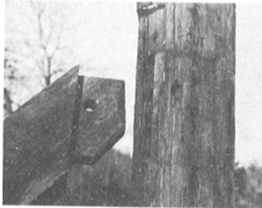
PLATE 430 The top of the diagonal brace was shaped to fit a mortise cut in the side of the vertical post.
