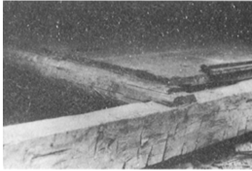
PLATE 453 The puncheon in place on the joist, which is resting on the main log sleeper.
