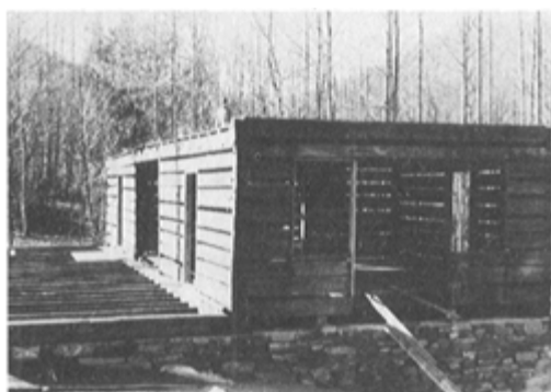
PLATE 416 The two logs that support the floor joists for the second floor are each 48 feet long—the longest hewn logs we have ever worked with.
