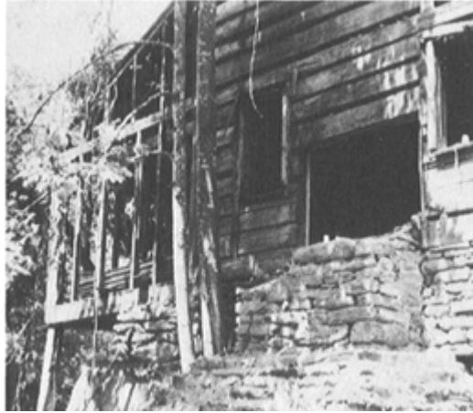
PLATE 396 The curved hand-cut rocks that once were steps are visible, stacked around the base of the chimney to help support it when years of rain finally washed the dirt out from under its corners. At the far left side of the photo, the end of room G is visible, supported by a post to keep it from collapsing before we could dismantle it. According to both Moot and Mitch, the bank visible under the room was not cut out by hand but was formed as the clay was eroded away from the house by rain.
