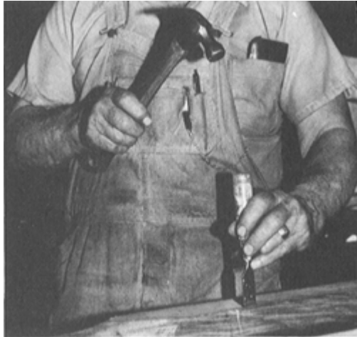
PLATE 301 The mortises are cut in the top of the front axle for the hounds ...
