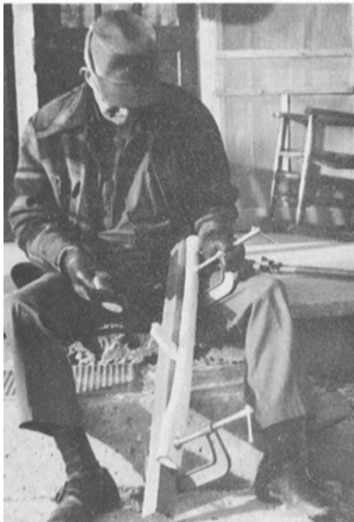
PLATE 469 When the handle is rounded off and shaped to roughly the correct dimensions, Frank clamps it at either end to a block of wood. Then he slips a wedge under the curve,
