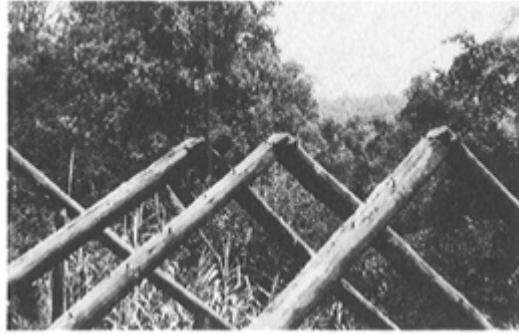
PLATE 398 In the kitchen addition, H, the rafters were round poles, lap-jointed and pegged.
