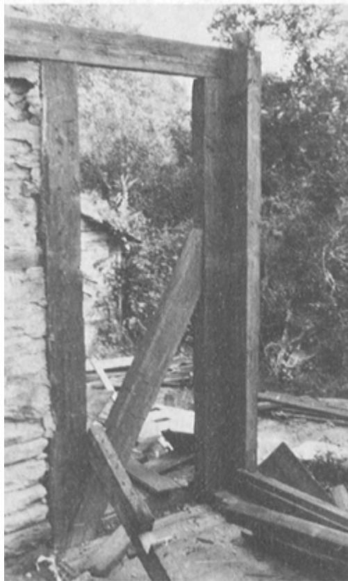
PLATE 401 The corner post beneath this point was supported by a diagonal brace ...
