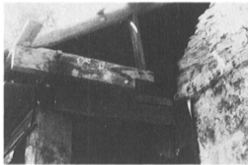
PLATE 399 When the kitchen was removed, an elaborate piece of mortised and pegged work was revealed, supporting the roof line for the dining room, F, at a point where F and H had joined around the kitchen chimney.
