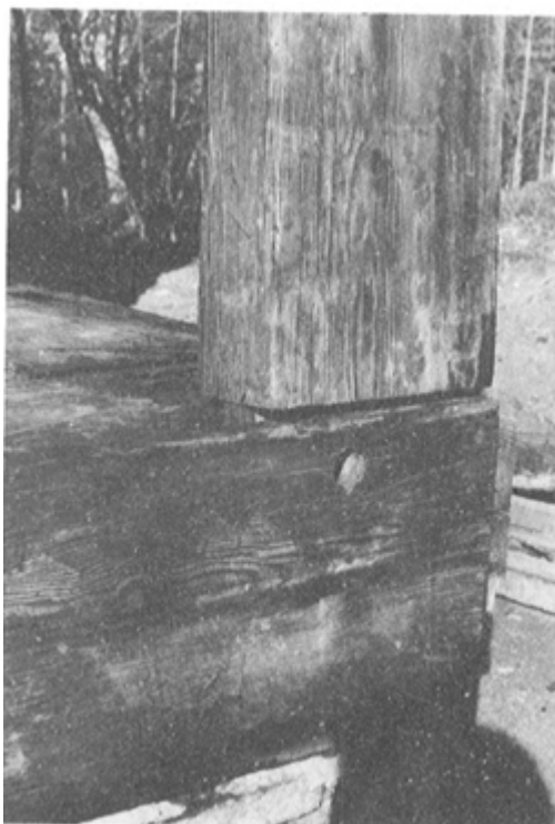
PLATE 428 The vertical corner post was fitted back into its mortise, and its diagonal brace was replaced and pegged.
