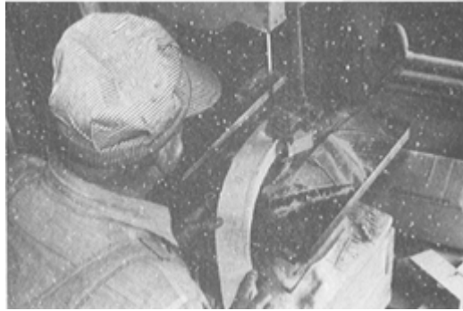
PLATE 239 When the felloes are outlined, he cuts them out on his band saw. Blacksmiths used to have to do this with a felloe saw (See Foxfire 2 ).
