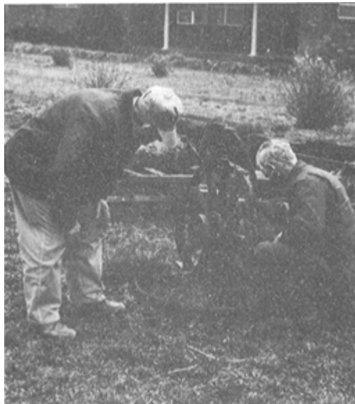
PLATE 268 Jud is now ready to make the axles and mount the thimbles, or spindles, and bearings, also called “boxing,” on their ends. Concerning the terminology, Jud says, “When we’d go to the store for these parts, we’d order ‘spindle and boxing’ for a wagon.” He salvaged the thimbles and bearings from an old wagon ...
