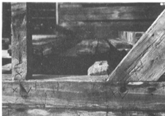
PLATE 432 The wall studs, diagonal braces, and sills were coded with Roman numerals by the original builders to show where each piece fitted.
