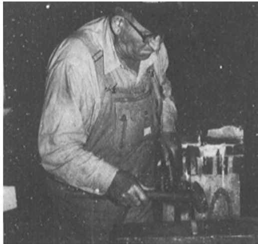
PLATE 209 Jud fashions the inner bands from quarter-inch by three-quarter-inch steel. Using a rawhide string to obtain the circumference of the hub where the band will go, he cuts them just short of the exact length they need to be. Then he scarfs their ends for forge welding. When scarfed and welded, the band will fit tightly around the hub.
