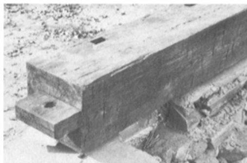
PLATE 424 A pegged mortise and tenon joint held the sills together at their corners. A mortise was also cut into the top of the corner to hold the base of the vertical corner post.
