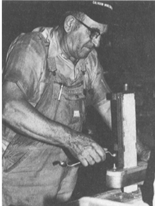
PLATE 315 He bolts one end of the metal strip that wraps the stake into the top of the bolster ...
