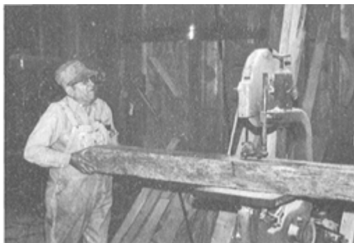
PLATE 270 Next he measured and sawed out the new axles from seasoned oak timber.
