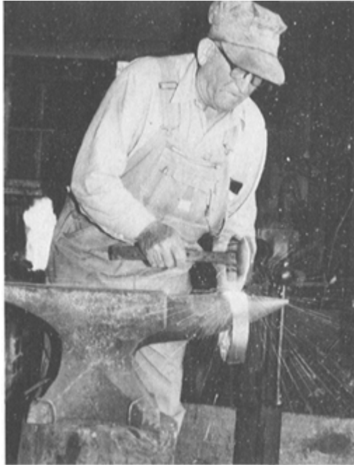
PLATE 212 Now the outer hub bands, measuring three sixteenths by one and a quarter inches, are cut, rounded and their ends forge-welded together.
