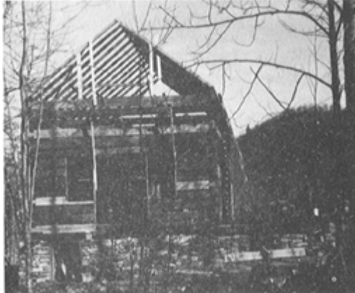
PLATE 422 The lighter-colored logs in the end of the building are new logs that had to be cut and fitted to replace rotten ones.
