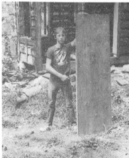
PLATE 454 Charles Phillips in front of Wig's log house, showing the underside of a puncheon board, this one made of poplar.
