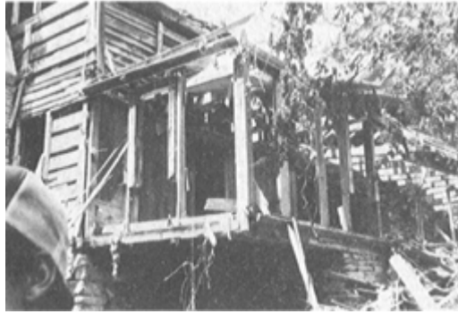
PLATE 394 The porch beyond rooms A and C had collapsed, so we began by removing the rotten debris and then tearing the siding off rooms A and C, which had been added to the original house in the 1920s.
