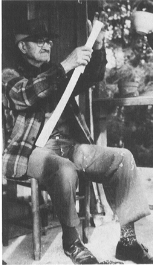
PLATE 475 Finally he sands the whole handle so that it is completely smooth. Then he greases it thoroughly with linseed oil to help waterproof it and preserve it and keep it from cracking.
