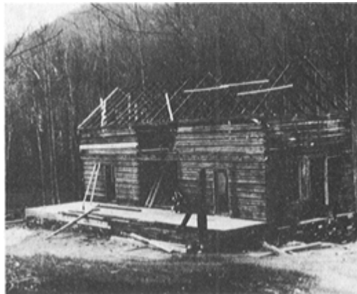
PLATE 422 The lighter-colored logs in the end of the building are new logs that had to be cut and fitted to replace rotten ones.
