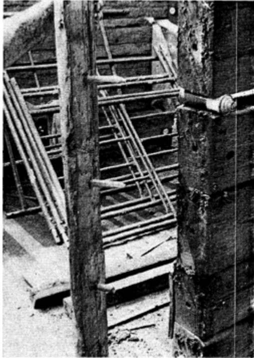
PLATE 407 Like the window frames, the door frames were also pegged into the wall logs—a technique that not only anchored the frames tightly into place, but also kept the wall logs separated and in line.
