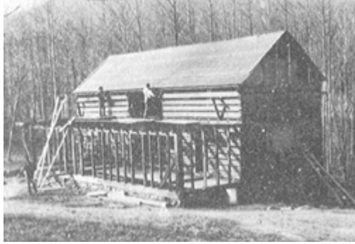
PLATE 449 Standing on the addition's ceiling joists are Frank Hickox (left) and Pat Shields, who supervised the moving and reconstruction. They are preparing to add the rafters for the addition. On the ground is Scott Shope, maneuvering for a camera angle.
