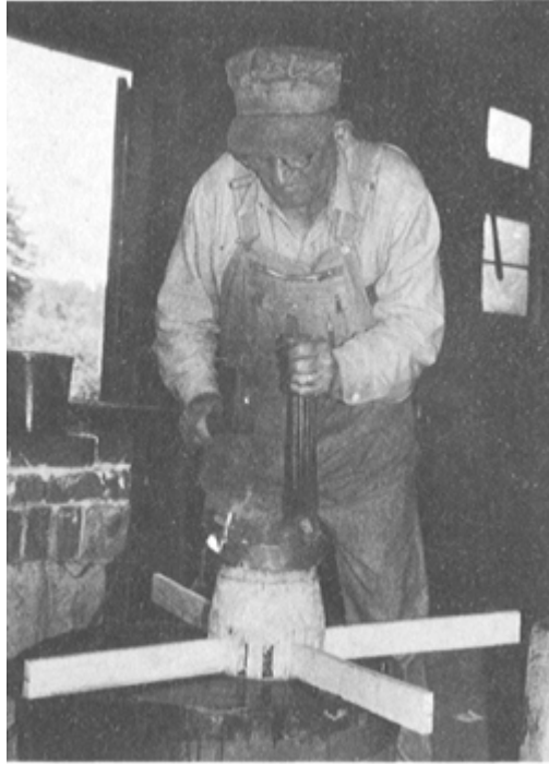
PLATE 216 ... and begins to drive the heated band onto the hub. As he does so the wood catches fire.
