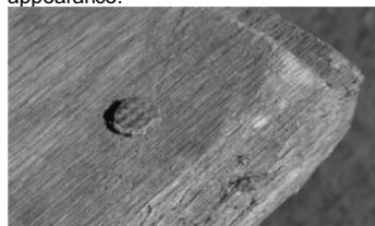
PLATE 150 A wooden mounting peg, driven through the shelf into the stabilizing block
