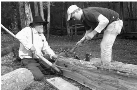
PLATE 142 Claud steadies the red oak log with a cant hook as Keifer drives in timber wedges, working on the second split.
