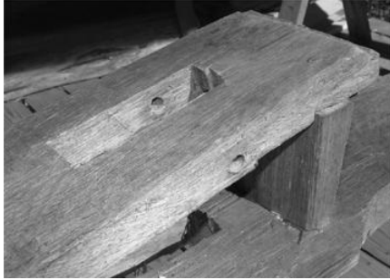
PLATE 151 Mounting holes for the dumbhead, drilled through the shelf
