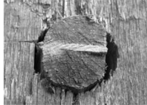
PLATE 147 The top of a leg in place through the bench, with a securing wedge inserted and trimmed flush
